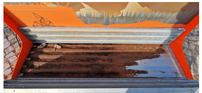
Fig 3- Retention tray full of dirt and debris. Drainage system of the BICCleaner clogged, lack of maintenance. (The in-built filter prevents clogging of the infrastructure pipes)
